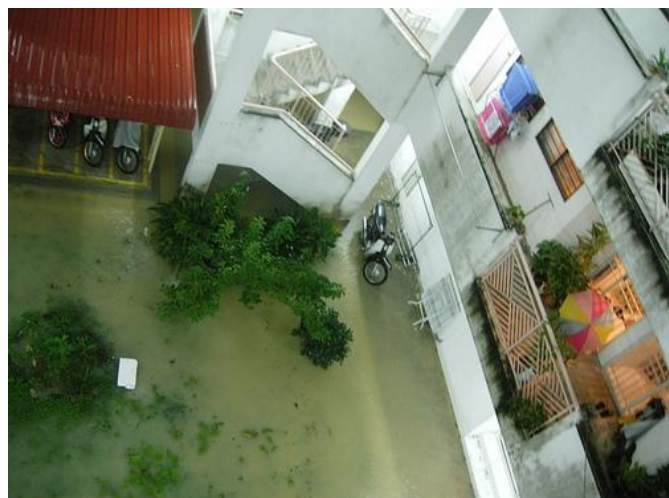
The water barely entering the ground floor apartment unit
